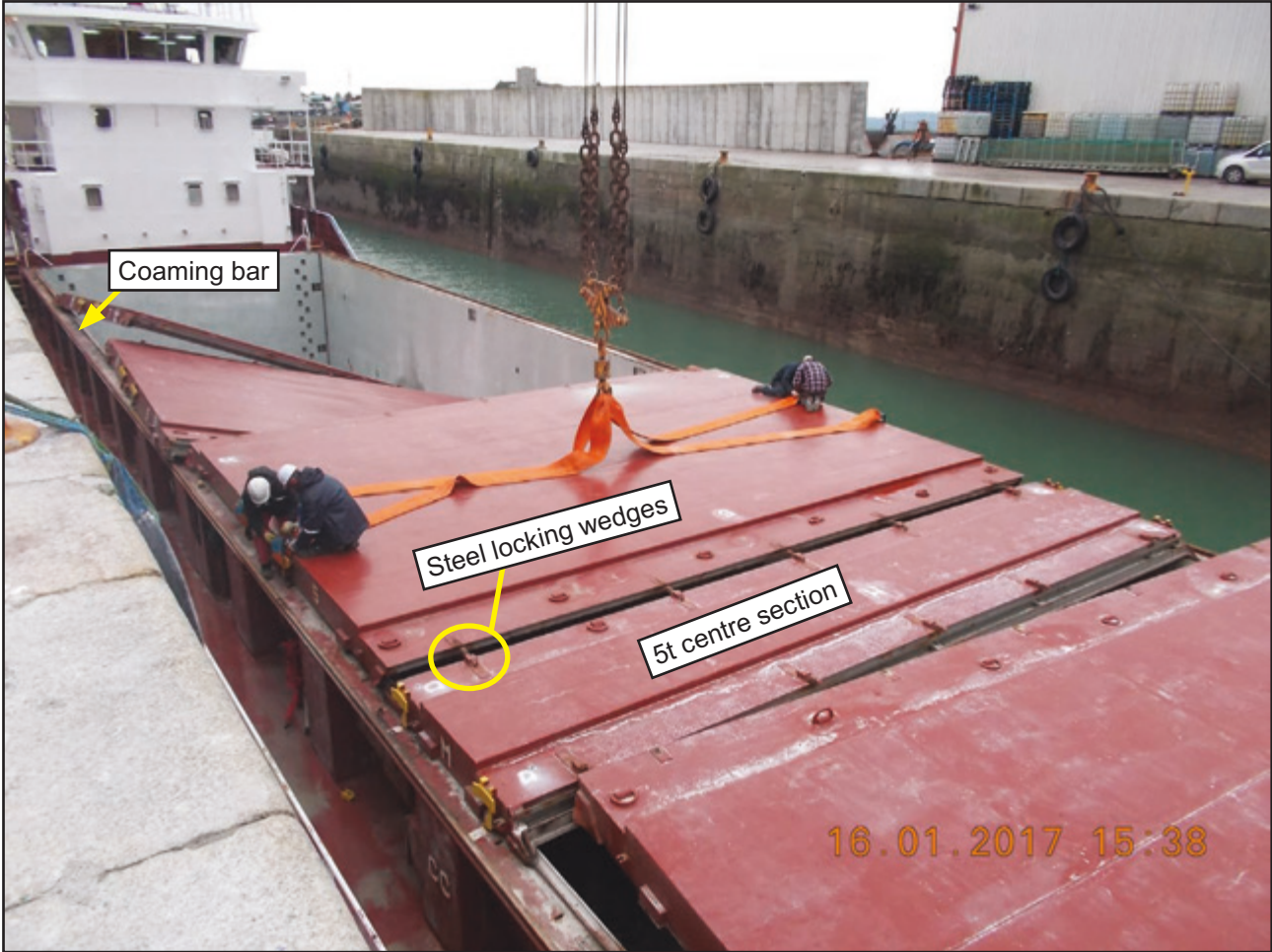
Figure 9b: Hatch covers undergoing temporary repairs
