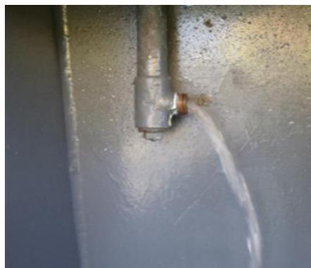
Figure 4: Non-return valve not fitted to the drainage arrangement
