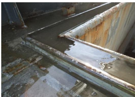
Figure 3: Overflowing drainage channels
