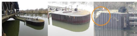
**Figure 121.** Left and center: Northeast protection cell for Rock Island Railroad Bridge. Right: View from across the river of damaged protection cell with impact location circled. SOURCE: CSX TRANSPORTATION.
