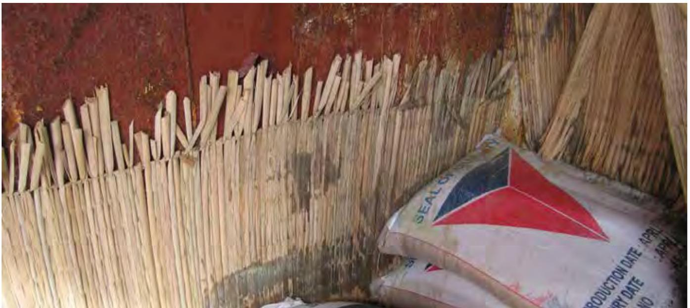
**Figure 1.6** | Bamboo mat dunnage along the ship sideshell has been stained through ship sweat. The bag adjacent to the dunnage has been stained through the migration of condensation through the bamboo mat into the bag.
