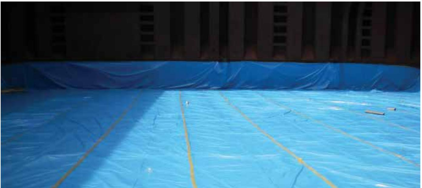
**Figure 3.6** | Kraft paper overlaid with plastic sheeting on the tank top. This continued vertically along the corrugated transverse bulkhead in background.
