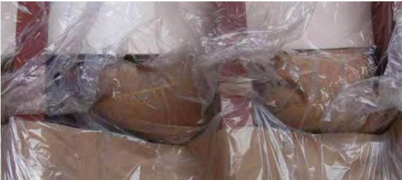
**Figure 3.17** | Saw dust in burlap bags is inserted at transition point between sideshell and top of hopper tank. Notice the Styrofoam sheets above and kraft paper beneath the bags is then overlaid with plastic sheeting.
