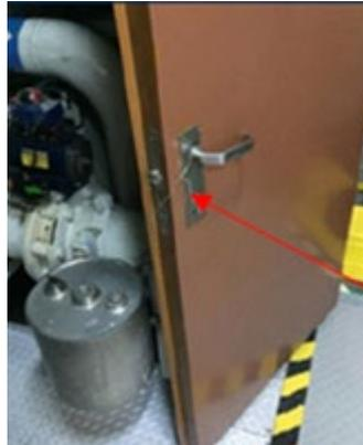
A fire door in the engine room was observed to be wired open – it was being kept open with piece of wire.
