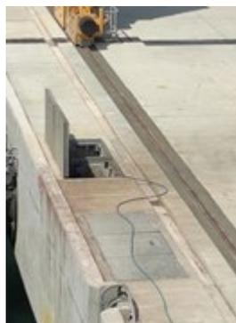
Two open hatches on the wharf in close vicinity to the vessel were observed and reported by vessel crew members. There were no barricades or safety signs installed, despite the potential fall hazard inside from 2m height. Following this intervention, the hatches were closed and locked by wharf service personnel.
