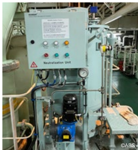
Ballast Water Treatment System found inoperable
