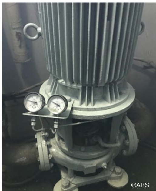
Fire pump running after repairs
