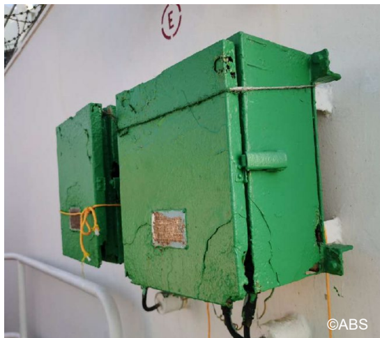
Electrical control boxes found broken
