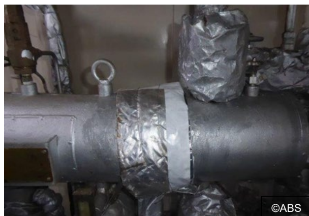
Fuel oil purifier flange isolated with band
