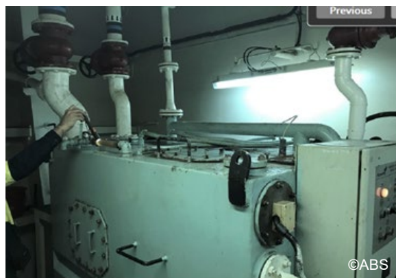
Sewage treatment system after repairs to air flow
