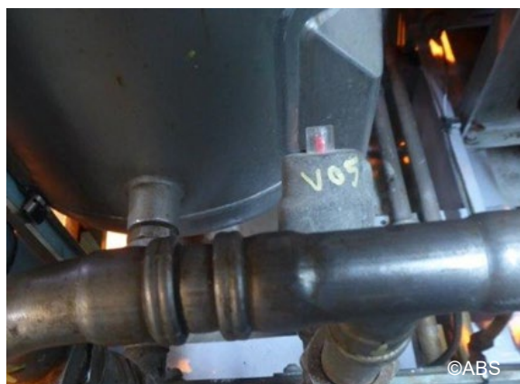
Oily water 3-way valve not functioning
