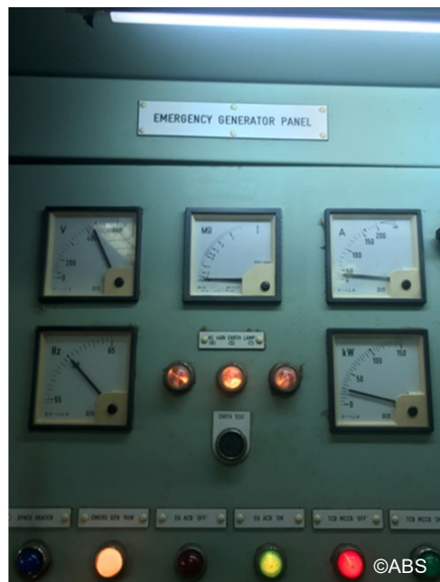
Emergency power auto start not functioning
