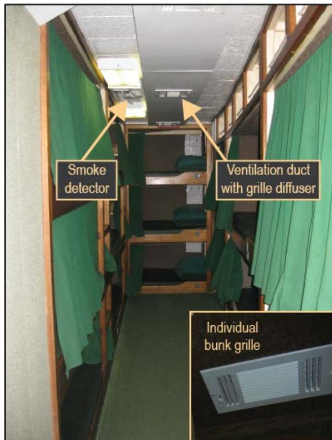
**Figure 16.** Port side of the *Conception's* bunkroom looking aft, with inset of grille/diffuser. (Source: M. Ryan; Inset: S. Landis)
