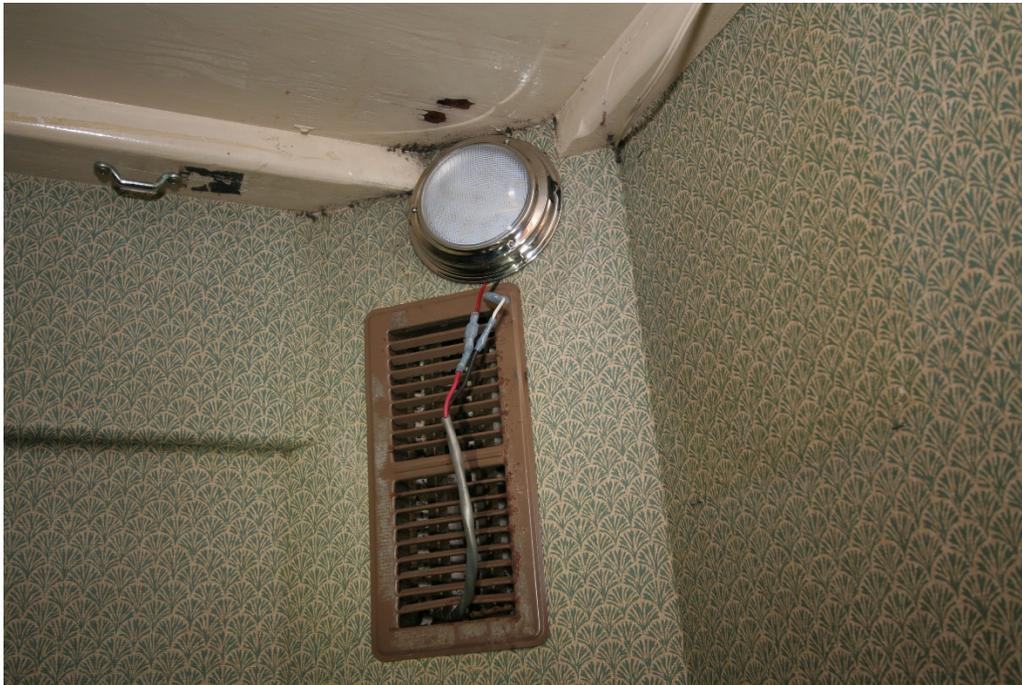
**Figure 23.** Power cable for lighting routed through ventilation grille in the *Vision's* bunkroom.
