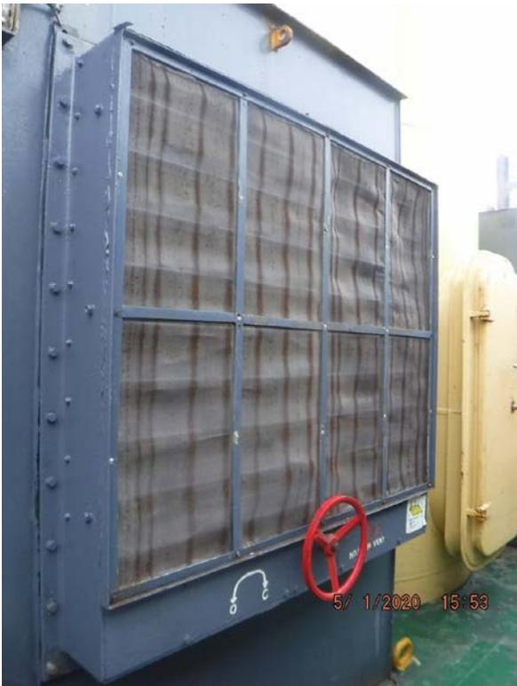
Figure 12: Mechanical ventilation with integrated closing damper (photo courtesy of OLDENDORFF CARRIERS GmbH & Co. KG.)
