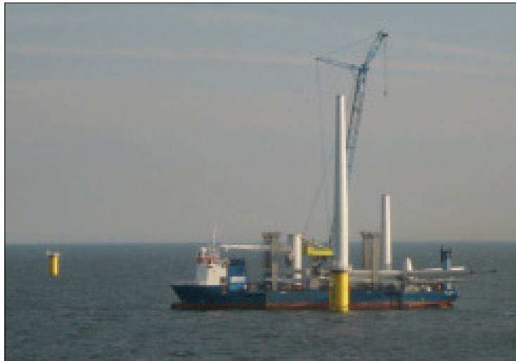
Wind turbine installation vessel (note the large crane)
