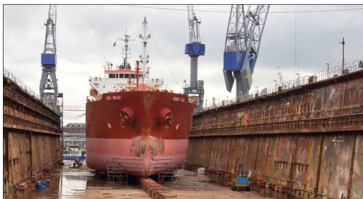
Dry dock & ship repair facility
