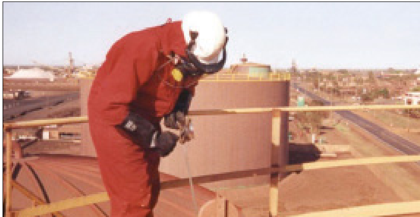
Measuring a chemical shore tank with a conventional tape and bob (Note the protective PPE)
