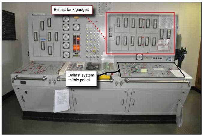
Figure 24: Ballast system control panel and tank gauges
