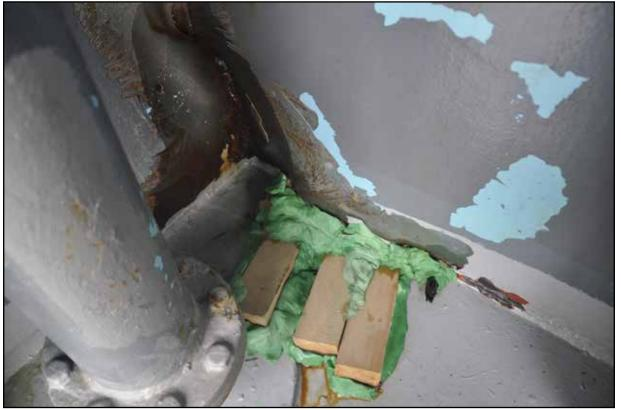
Figure 9: Temporary patch applied to shell damage by salvors
