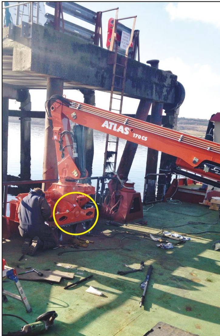
**Figure 17:** Crane installation showing inboard box section (circled)
