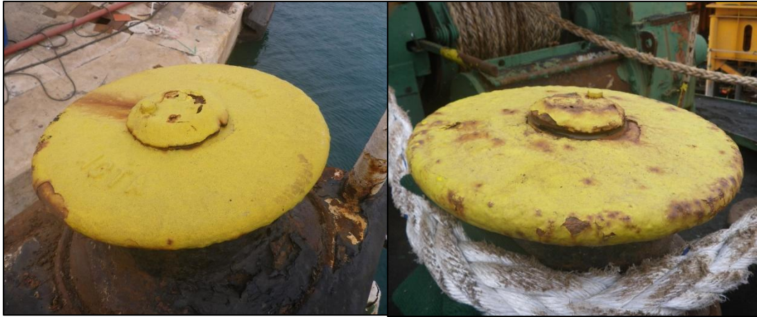
Figure 16: Other rollers at the aft mooring station
