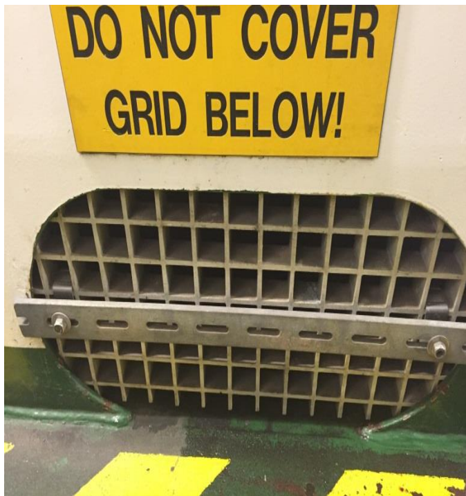
Fig 8: Vehicle deck drain
