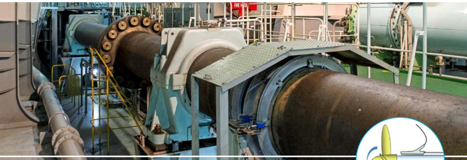
DNV GL has revised the main class rules for single stern tube bearing installations and now offers new optional shaft alignment class notations.
