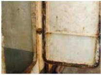
Figure 2: Poorly maintained access rubbers
