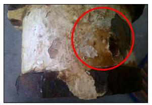
Figure 8: Layers of paint and corrosion
