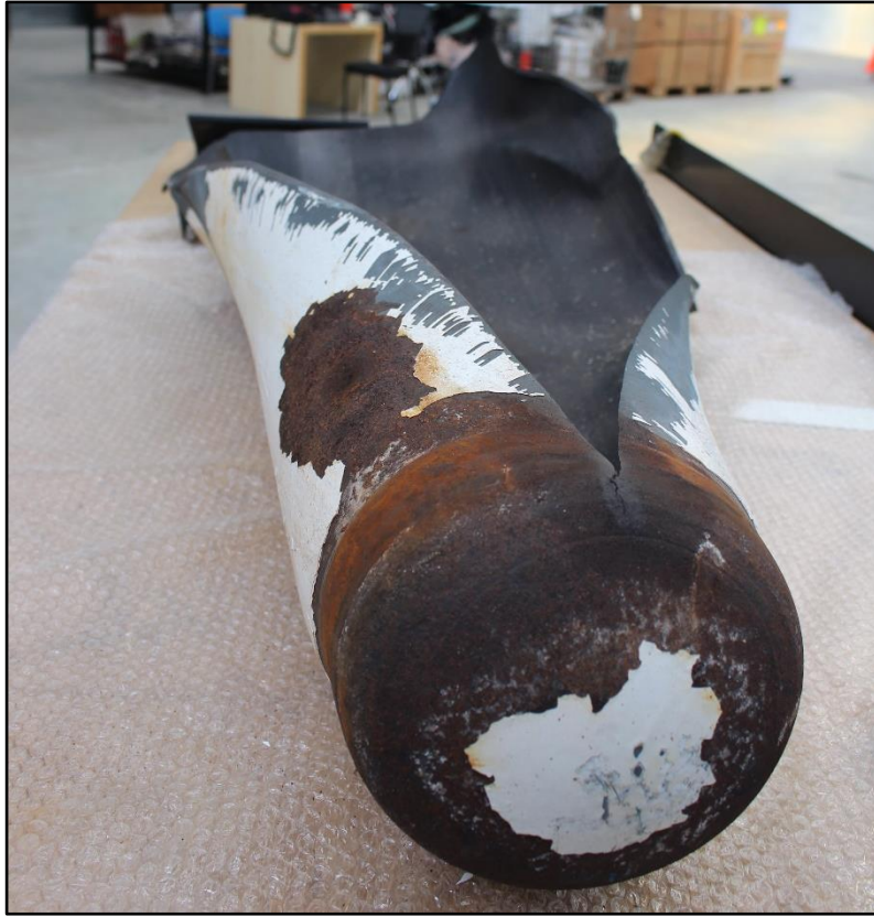
Figure 11 Area of corrosion near the bottom of the failed cylinder
