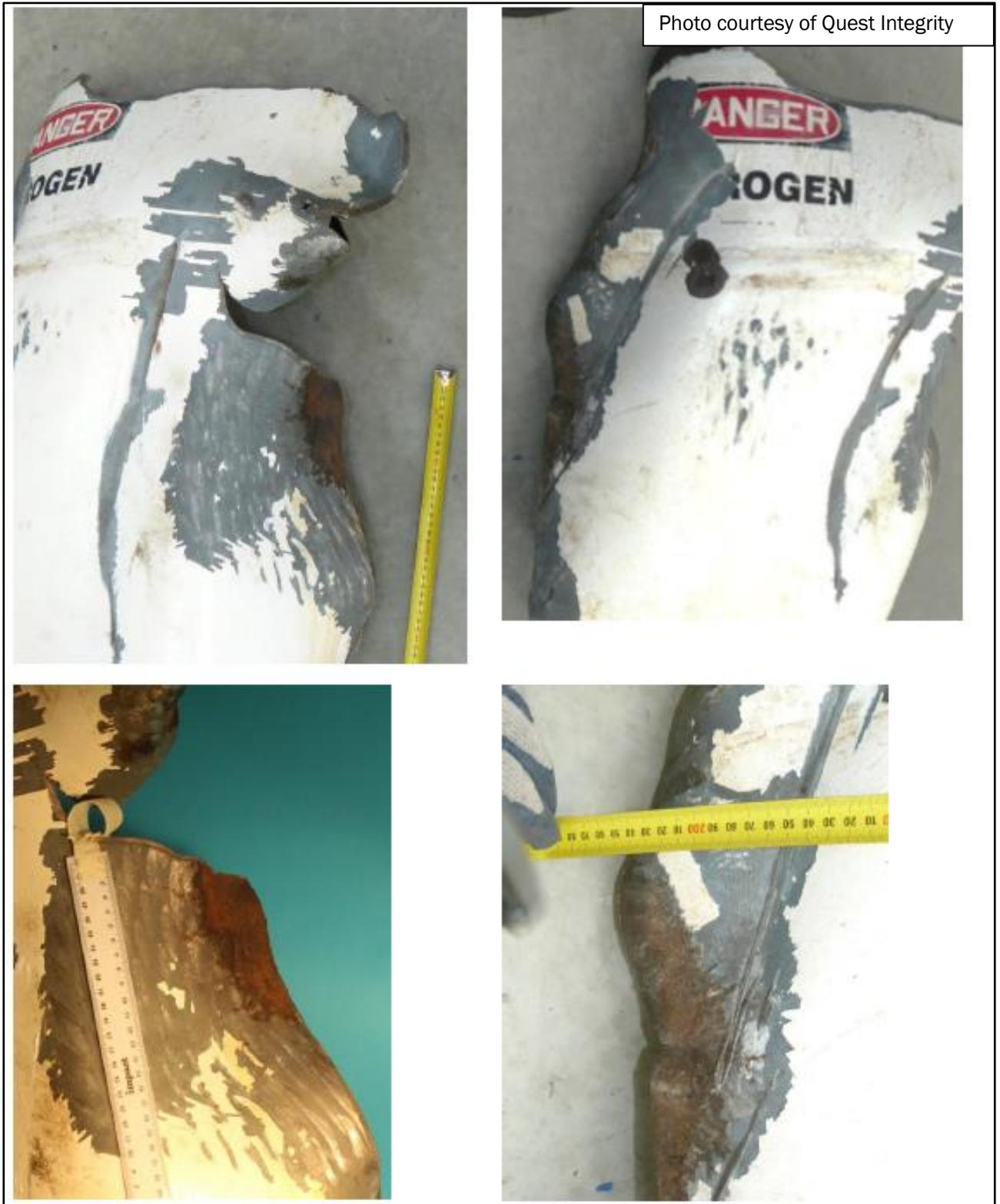
Figure 10 Area of corrosion at the area of initiation of failure
