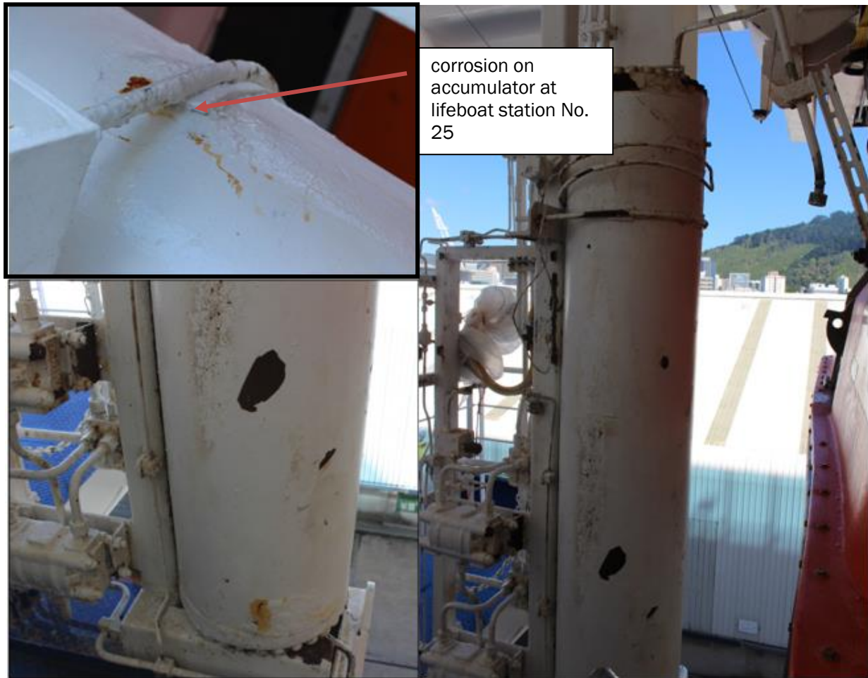
Figure 14 Corrosion on accumulator
