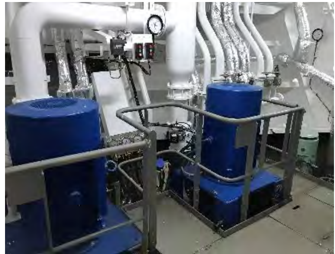
Figure 3.5 | Seawater pumps for scrubber system in engine room
