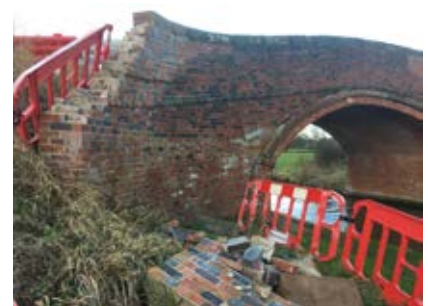
Above: Golden Nook Bridge vehicle damage
