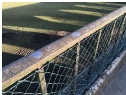
Above: Repairs to ironwork, Chirk Aqueduct
