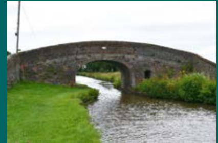
Above: Roundthorn Bridge before repairs
