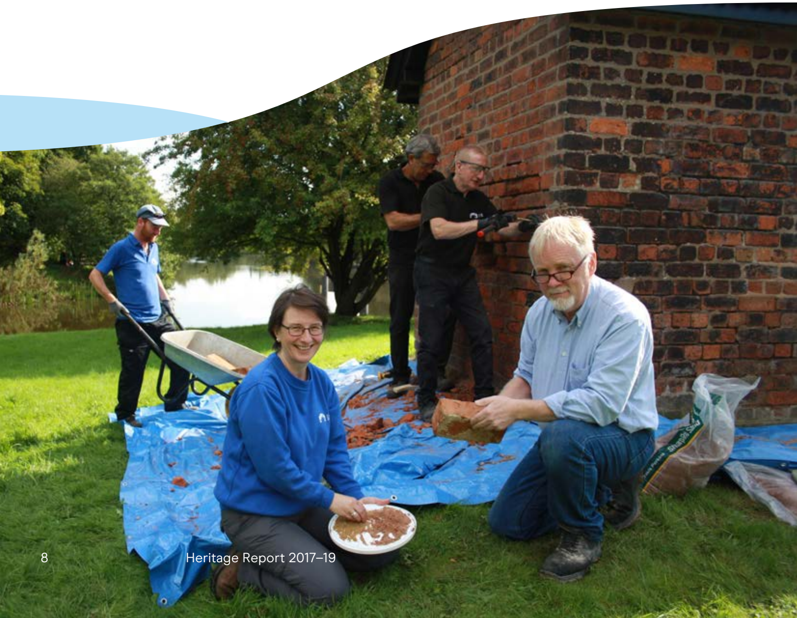
Below: Bridge-keeper's hut repairs team
