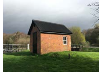
Above: Bridge-keeper's hut restored
