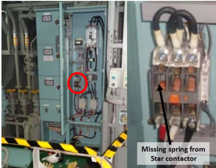
Figure 5: IG scrubber pump starter contacts and the missing star contactor spring.
