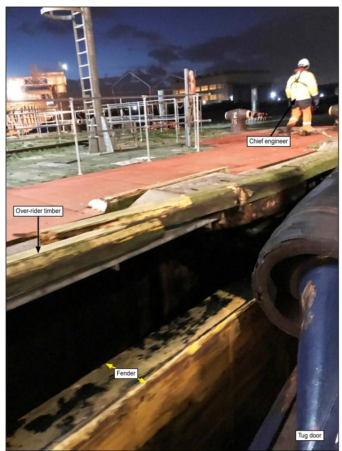
**Figure 4:** Chief engineer on north oil stage about to release the head line (photograph taken by a crew member to record damage caused to over-rider timber)
