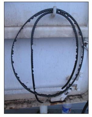
Figure 9: Broken belts of the emergency generator fan
