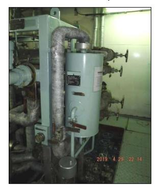
Figure 6: Compensation damping tank
