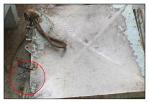
Figure 16: Rubber strips wrapped around securing points and securing dogs lying on the side
