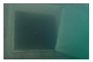
Figure 8: Hatch on port side freeboard deck in way of the fish hold found open
