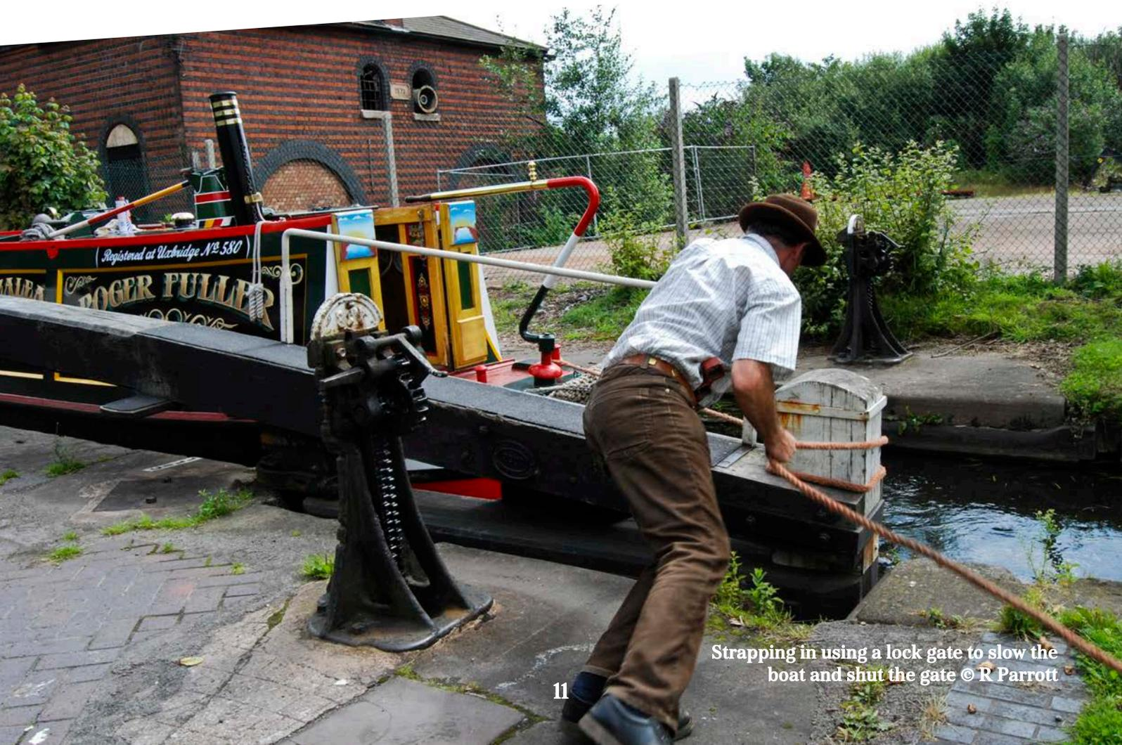
Strapping in using a lock gate to slow the boat and shut the gate © R Parrott
