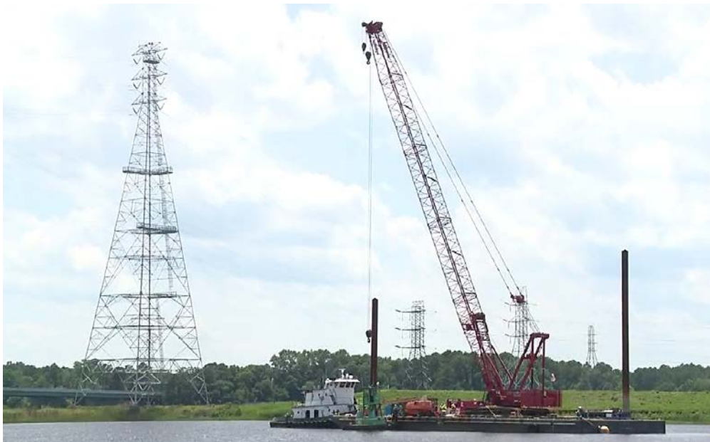
Towing vessel Goose Creek and crane barge U1510 spudded down in Chesapeake, Virginia, after the accident.
