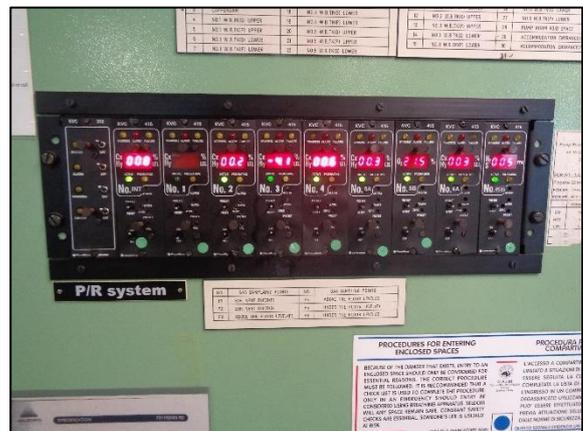
Figure 11: Display panel of the fixed gas detections system
