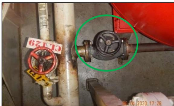
**Figure 15: Suction valve (circled in green) of the starboard bilge of the pump room**
