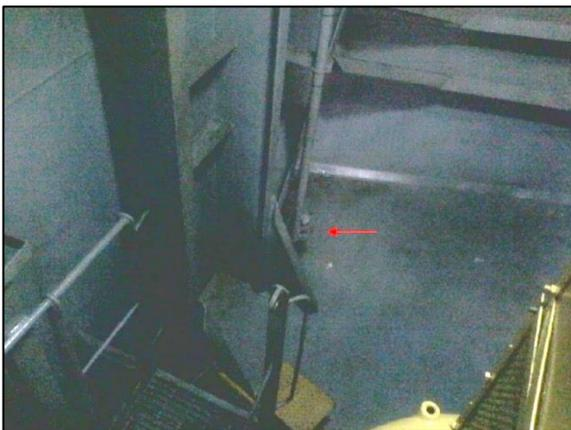
**Figure 4: Port side bilge alarm sensor (red arrow), as seen from the lowest pump room gratings**
