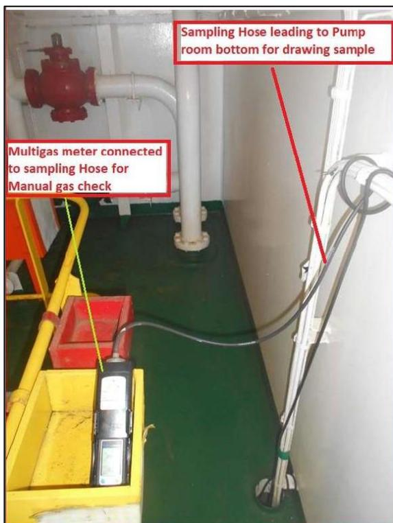
Figure 12: Personal multi gas detector placed at the pump room's entrance
