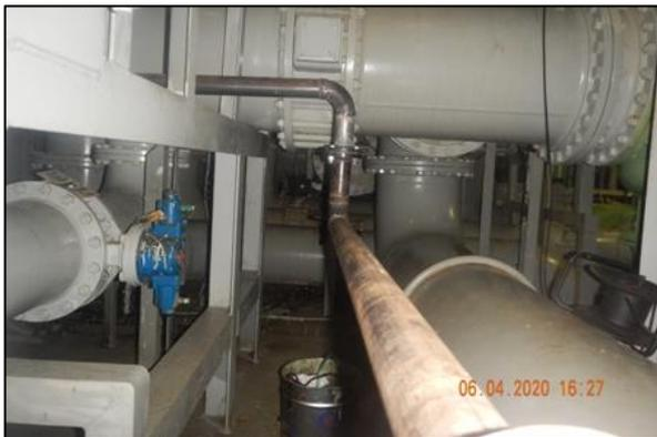
Figure 19: Modified arrangement for stripping of the AUS drain tank
