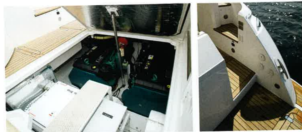
Access all areas: the engine bay is about as shipshape as you will find, while deck safety shines out
