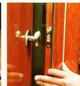
Anti-rattle seals have been added to the door frames
