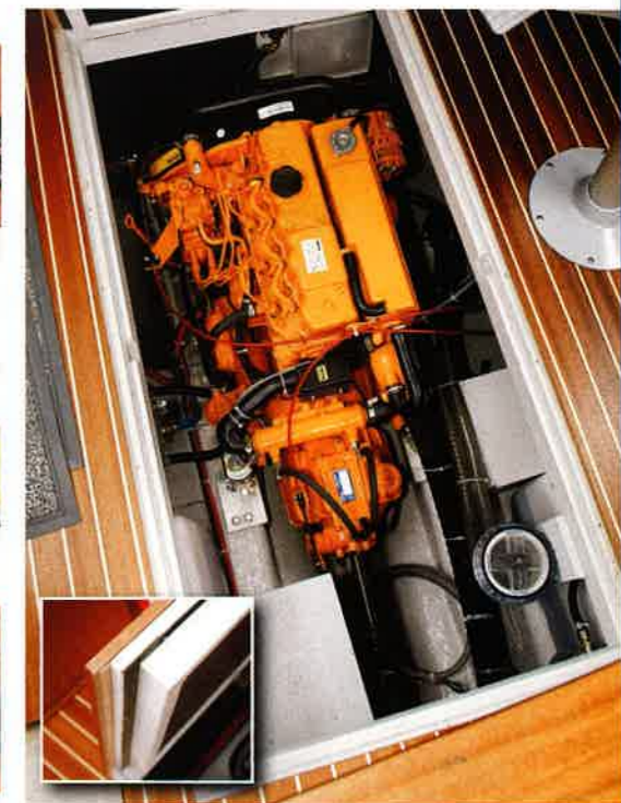
above Engineroom hatches are well soundproofed.
