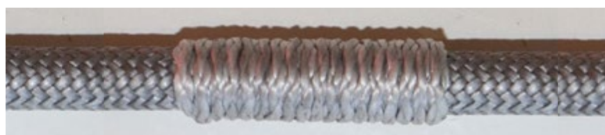
Figure 2: Whipping on lifeline rope for chafe protection
