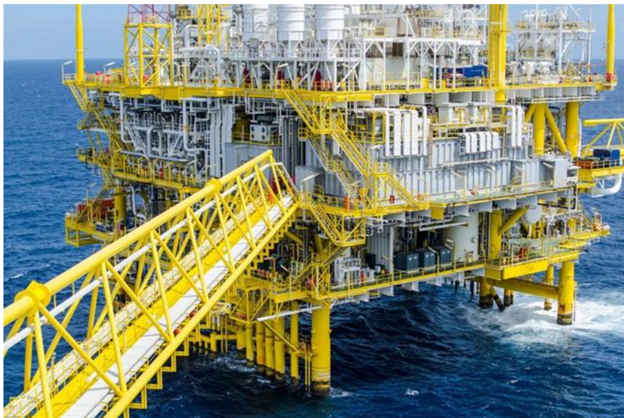
Figure 4. Bridge between two platforms
