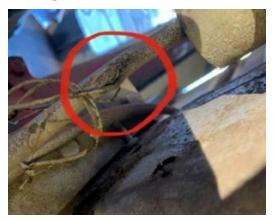
During a washdown of a vessel's cargo hold a crew member noticed arcing from around two electrical cables near the cargo hold light. Upon closer investigation he noticed a piece of tie wire connected to the cables was glowing red. The crew member immediately stopped hosing down and turned the water supply off and notified the ship's electrician.
